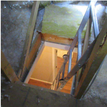
Image 3.11.3 - Entry to attic
